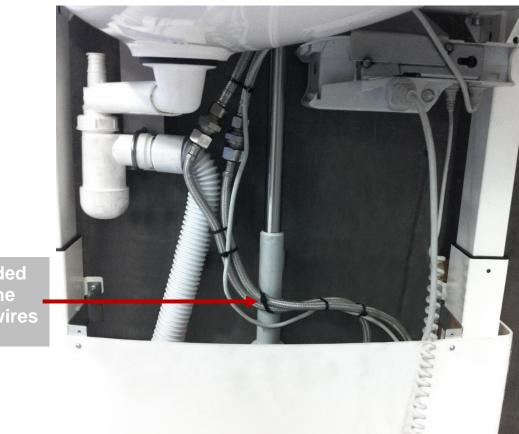
Recommended fixation of the hoses and wires
