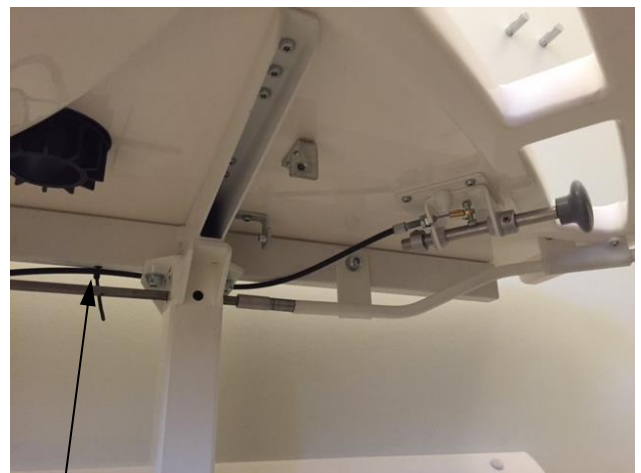
Washbasin viewed from below with wire fastened with strips.
